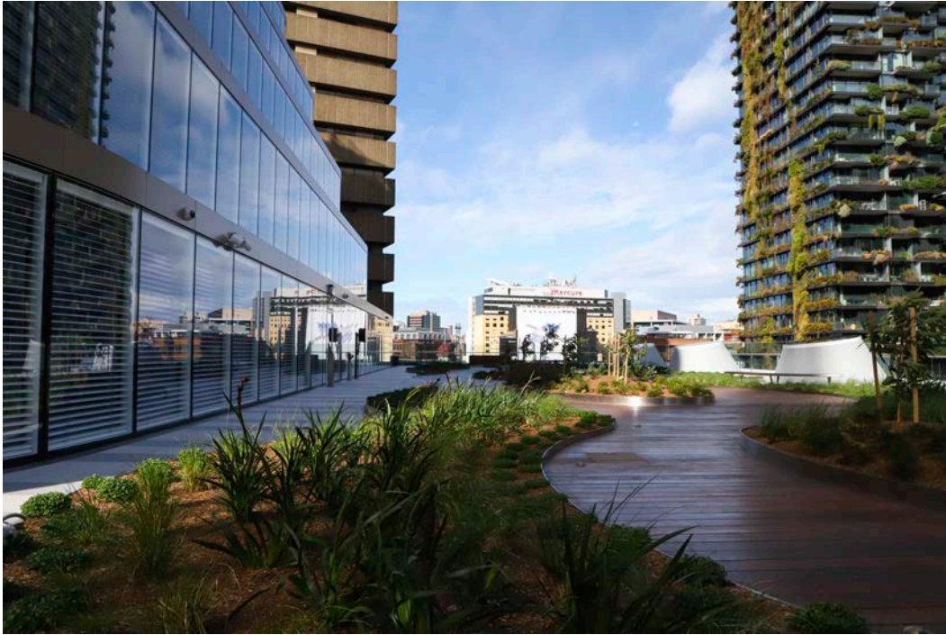
Library terraces. Level 8.
